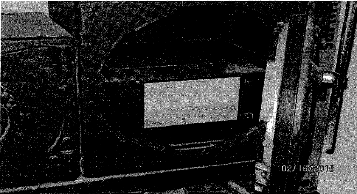
Figure No. 6 Date Taken: 2-16-15 Facility: Manuel F.L. Guerrero Administration Bldg. Description: Fluorescent lamps & possible asbestos containing safes located in the former Treasurer of Guam office
