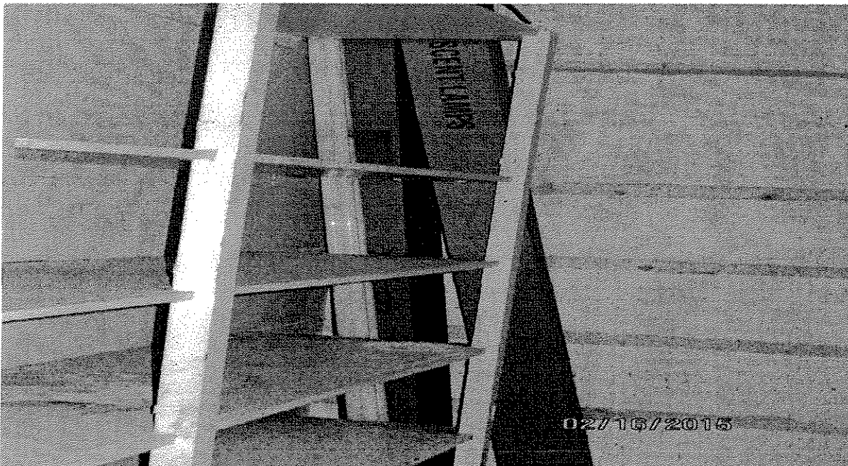
Figure No. 12 Date Taken: 2-16-15 Facility: Manuel F.L. Guerrero Administration Bldg. Description: Fluorescent lamps located in room #260 former DOE offices 2 nd floor
