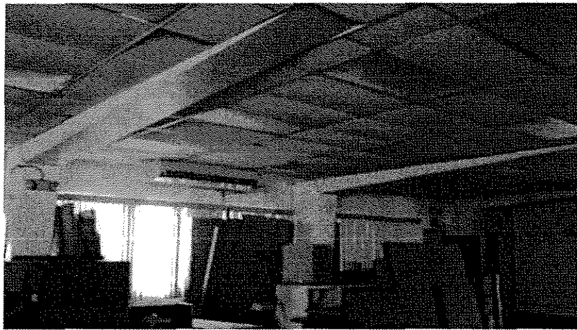
DOA First Floor AC Ventilation (no power for testing)
