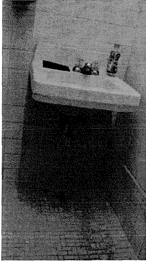
DOA Director Office Rest Room Lavatory
